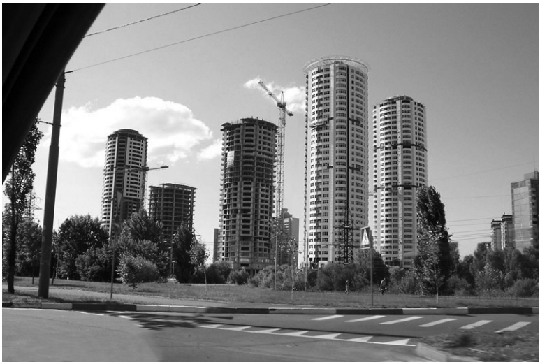
Figure 10: New apartment construction, Kyiv.
