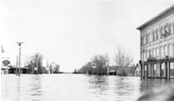
Figure 19 Main Street Emerson during 1950 Flood Source: RM of Morris (2018)
